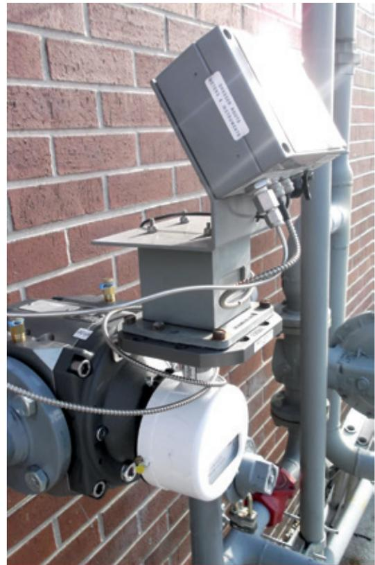
special product characteristics, such as for example the RABO-ID with mechanical index drive for generating impulses for American gas volume correctors (see Fig. 1), and on the other, the necessary product certification in accordance with the American standard ANSI B109.3 for rotary gas meters.
