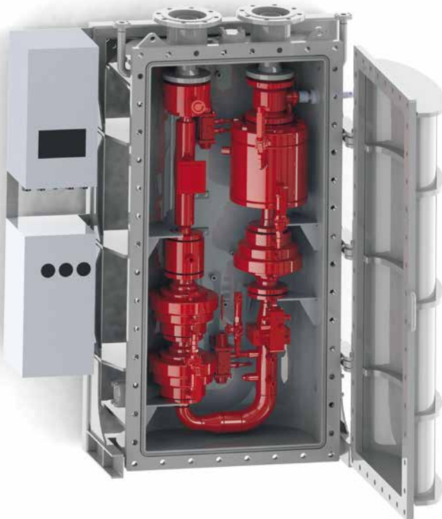
Fig. 2: Shut Off Valves HON750 in Ship Control Section in a Gas-tight Enclosure
