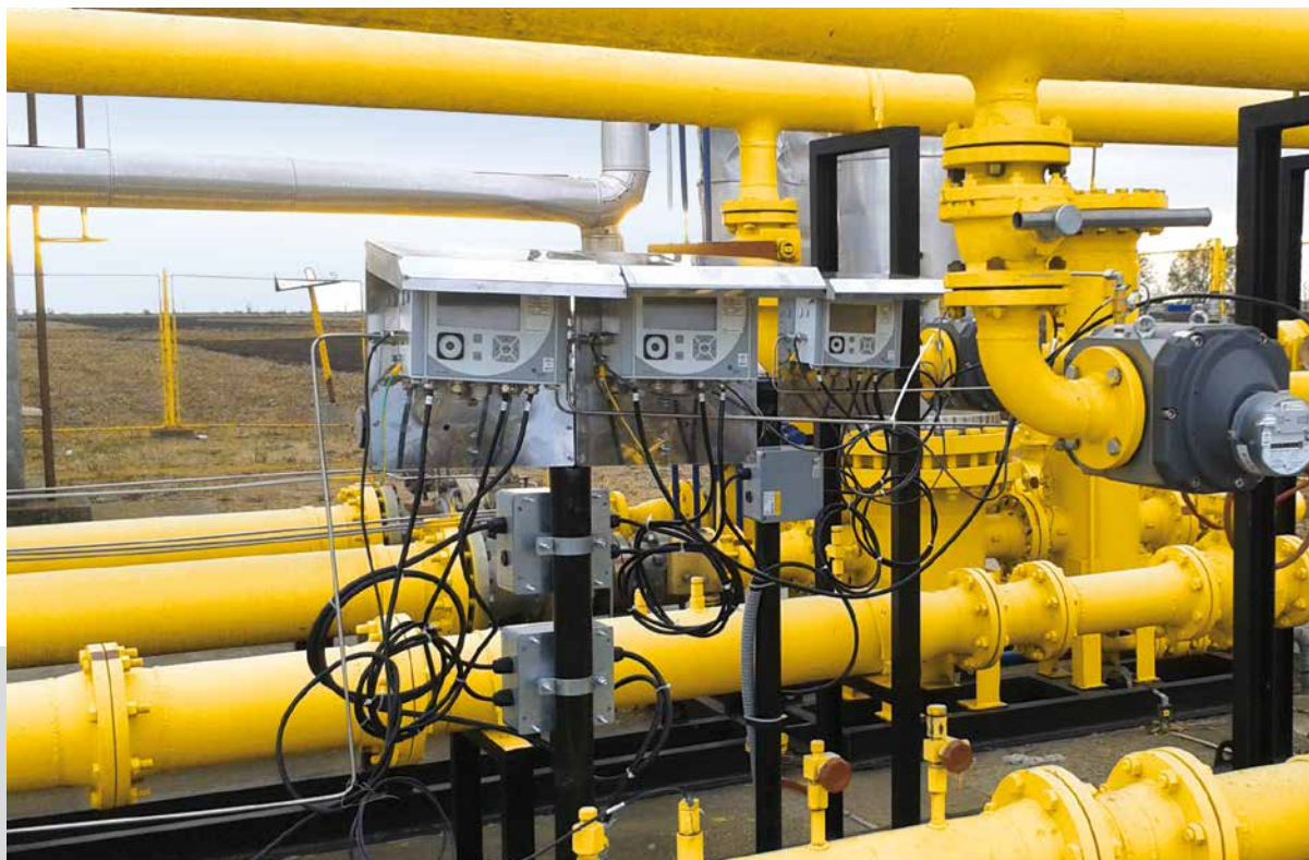
Fig. 1: EK280 in Station Operated by Srbijagas
